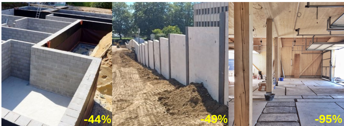
Lot 1 Constructions souterraines
