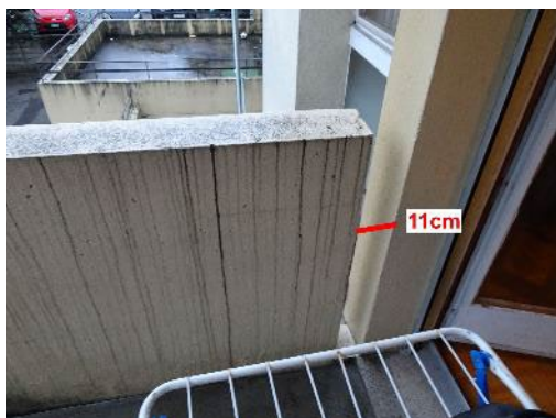
Parapet balcon Interstice conforme
